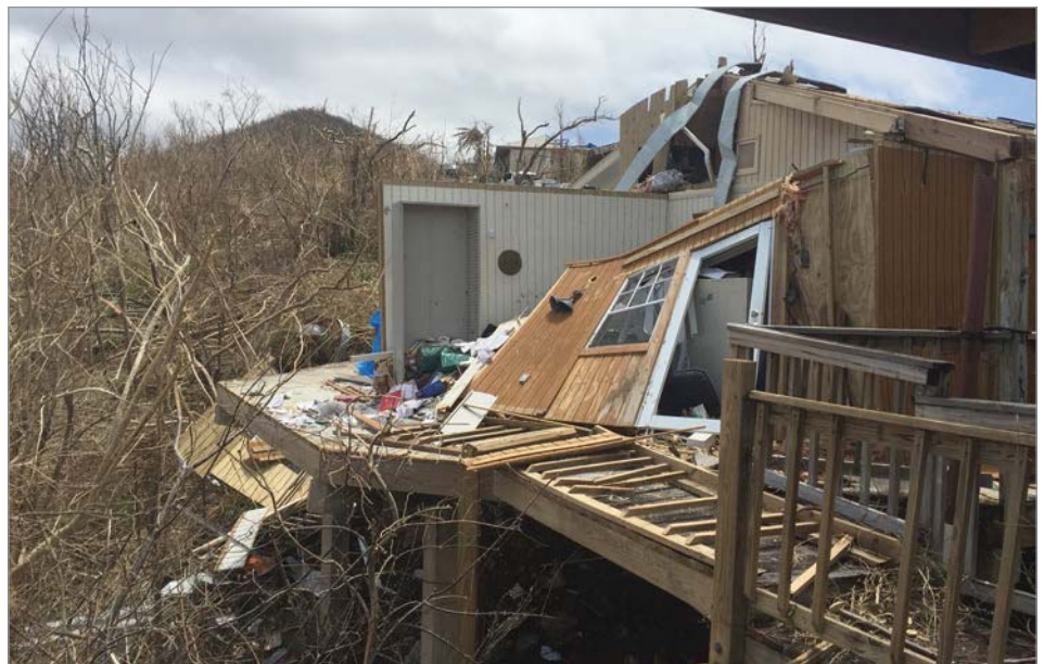
The remains of the NPS building adjacent to Caroline's that housed Chief of Resources and Administrative support offices. Photo credit: Jeff Miller, NPS
